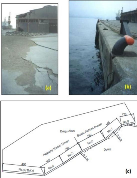
**Figure 1.** Damages due to the 1999 Marmara Earthquake on the blocky quay wall of Derince Port, (a) Traces of liquefaction in the backfill between the transit warehouse and the quay wall; (b) Seaward movement of the quay wall; (c) Horizontal displacement pattern determined after the earthquake [8].
